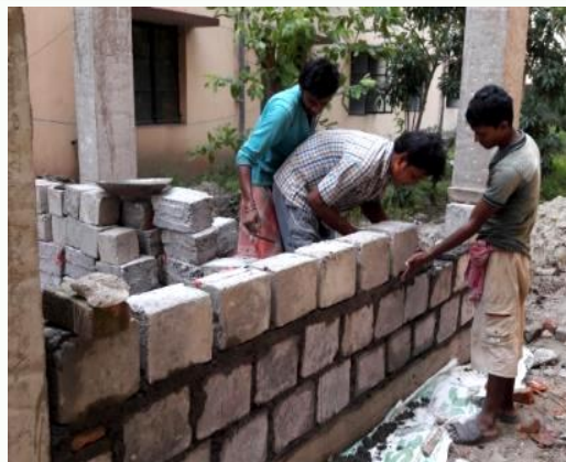
Toilet using Recycled Construction Materials
